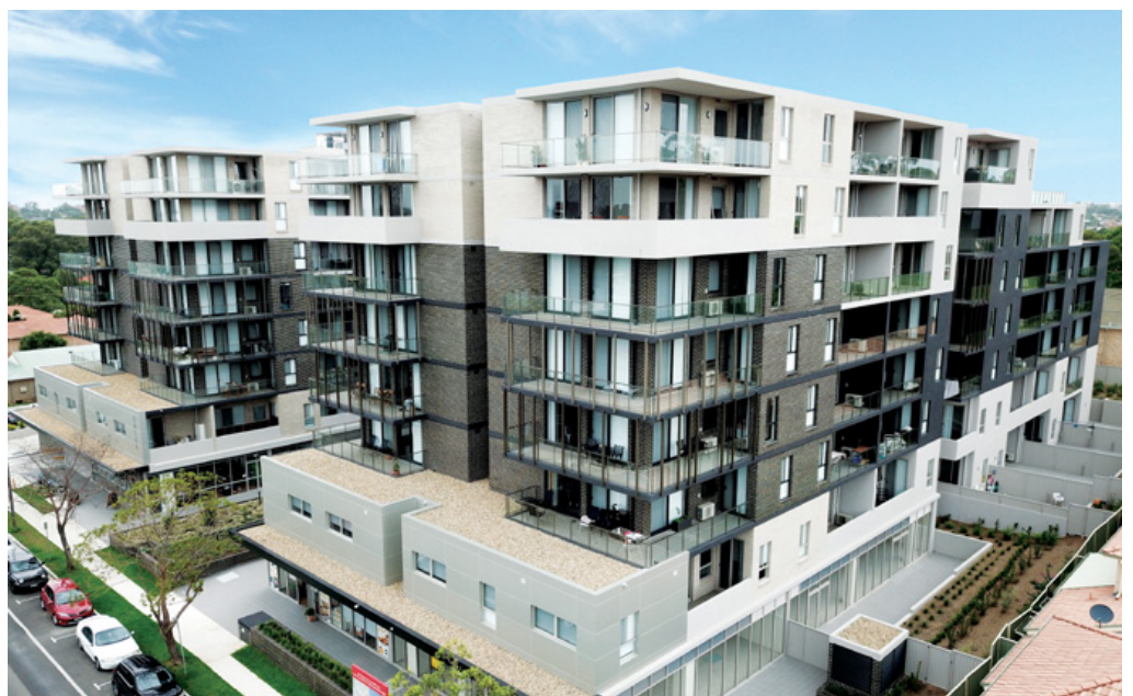
Omega Apartments, Kingswood NSW
